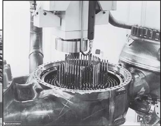
Special vertical 120 Inertia Friction Welder has CNC table to position space shuttle main engines for welding of injector posts. Superalloy injector posts are welded to space shuttle main engine. 600 posts per engine, 3 engines per shuttle.
